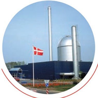
Power Plants, Diesel /gas engine (built by Wärtsilä)
